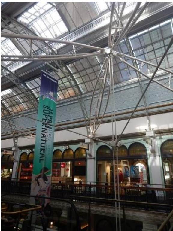
Fig. 7 – Steel suspension structure for new escalators southern end Second Floor
