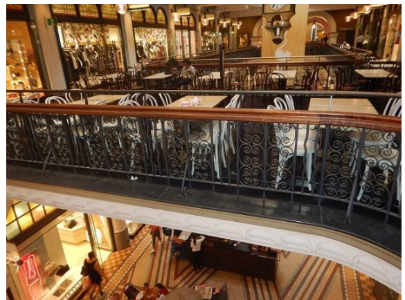
Fig. 12 - New BCA compliant glass and metal balustrade
